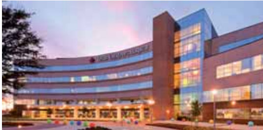
Texas Childrens Hospital, Houston_USA
