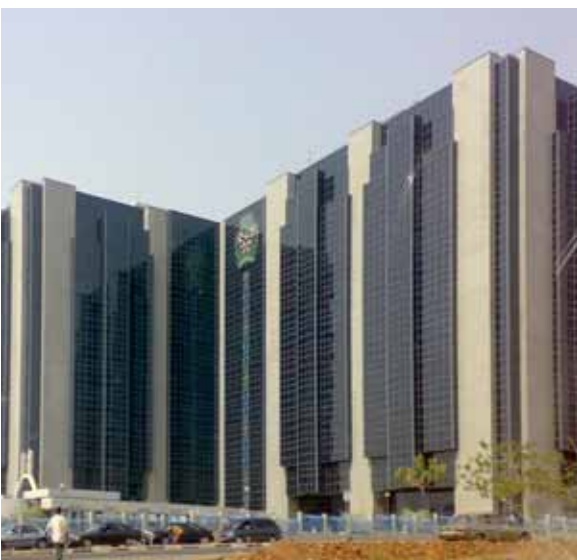
Central Bank, Abuja_Nigeria
