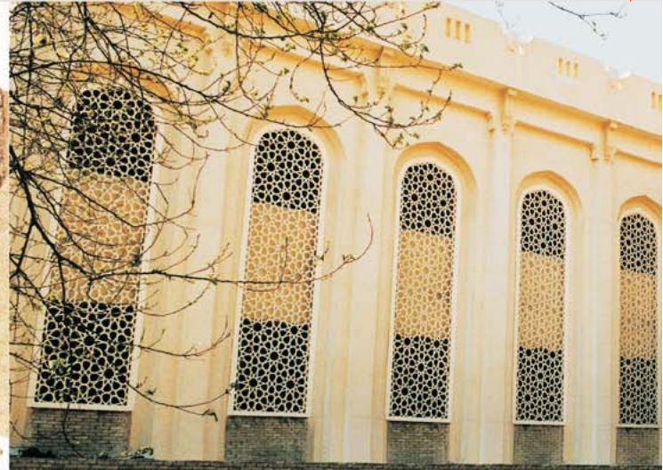
AMF Project University of Cairo Egypt
