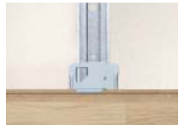
Push plank and block with clip.
