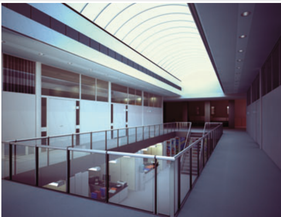
CONTINUOUS ROOFING Model of tunnel with reinforced aluminium profil
