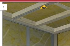
Install the first row of panels following the line. Remember that there must be a 10-mm clearance by all fixed structures. It is essential that the underlay is perfectly straight. Any unevenness in the framework MUST be corrected before installation.
