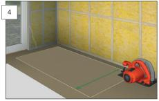
Measure and cut the first panel (panel width must be minimum 550 mm). Be careful with the panel's profile. When using a saw, place the panel with the foil facing
