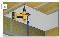
Panel row no. 2 . Cut the first panel in the second row of panels. The joint on the panels short side are staggered. Glue the profile, then click it into place.
