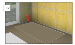
On the next panel, glue both the long side and the short end. The rest of the ceiling is installed. Tip! Place the ceiling support as close to the shortend profile as possible. The panel will easier click into place when using the tapping block.
